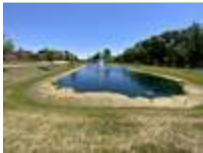
View of the stormwater retention pond
