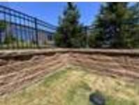
Fencing installed above the block retaining wall
