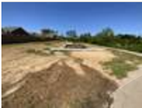
View of the stormwater detention basin
