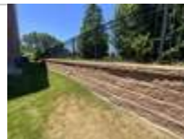
Typical view of the concrete block retaining wall
