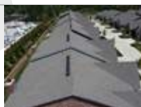
Typical view of the roofs
