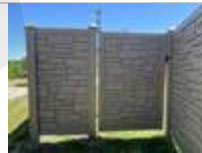
Vinyl fencing and gate
