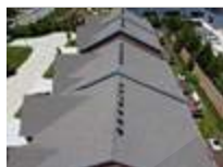
Typical view of the roofs
