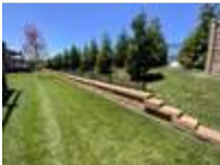
Fencing installed above the block retaining wall
